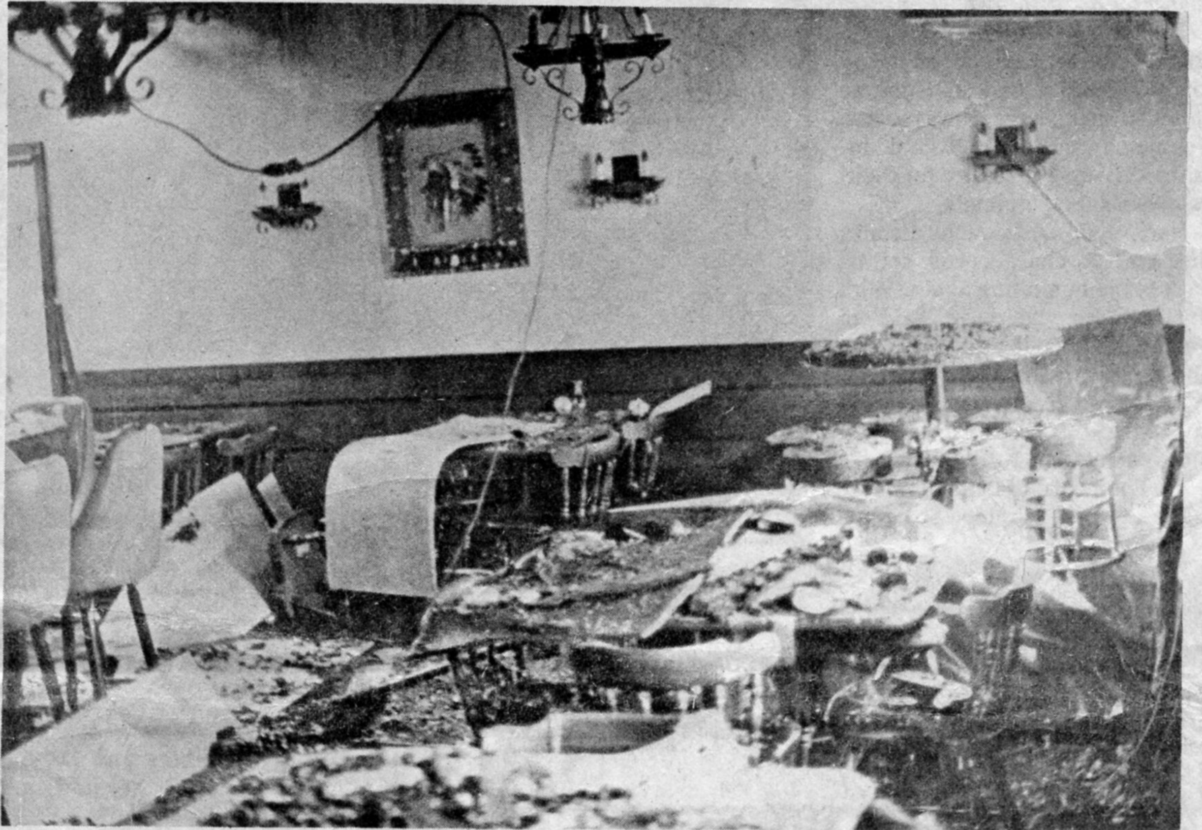
The Comeback Inn was also left in shambles after the flames swept through the commercial complex housing five city businesses. Edgerton TV Repair Service, in an adjacent building, also received smoke and water damage in the blaze.
