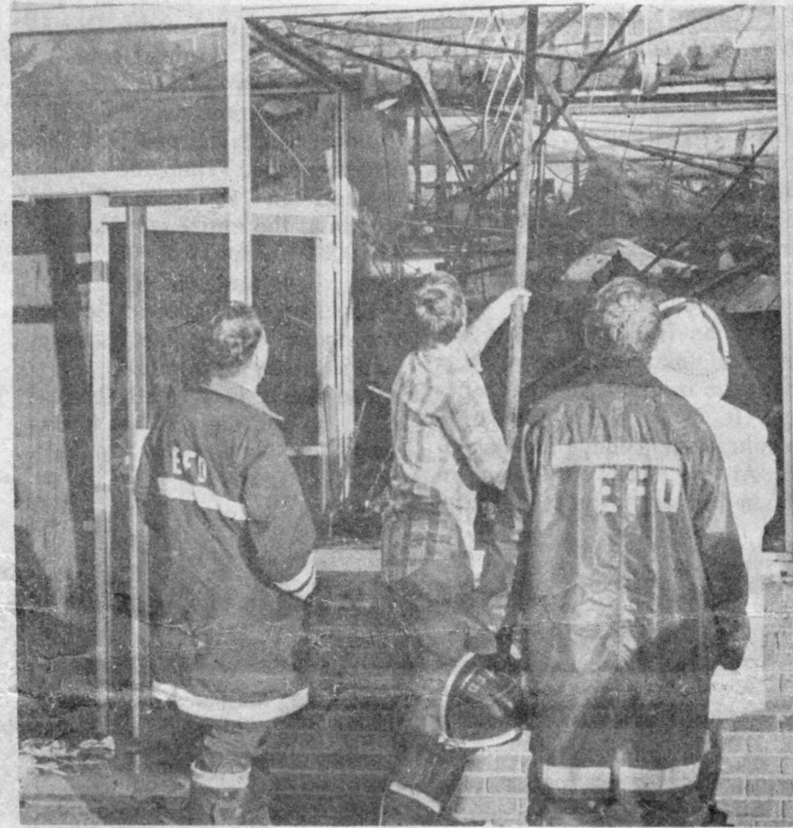
Edgerton firefighters struggled with the blaze that virtually gutted the Comeback Inn and the Dairy Queen Restaurant for nearly seven hours Monday morning.
